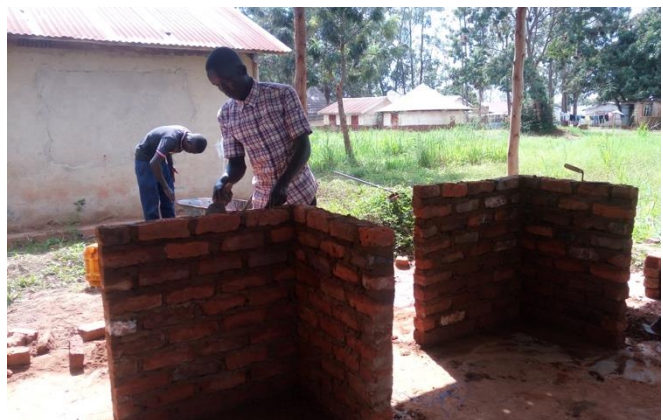
The trainees during their first practical lesson on making a return wall.
