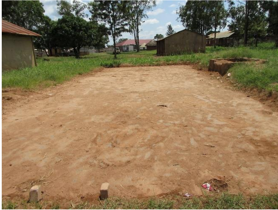
The location of the former training shelter for the Bricklaying and Concrete Practice class, which collapsed. This has delayed the practical classes for the current intake due to lack of training space.
