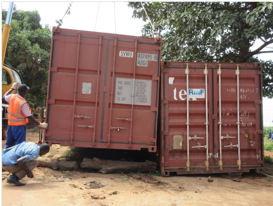
The container that was delivered at Panyadoli Health Centre III; beside it is a container that was delivered previously.
